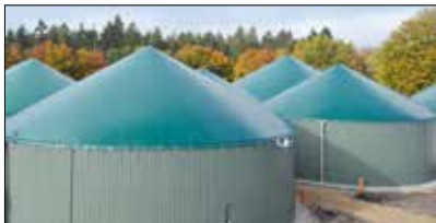
Biogas facility at Gut Hülseberg
